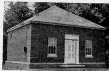
[Courtesy: Bell System Technical Journal.] Fig. 2. Auxiliary repeater station on New York-Philadelphia route.
